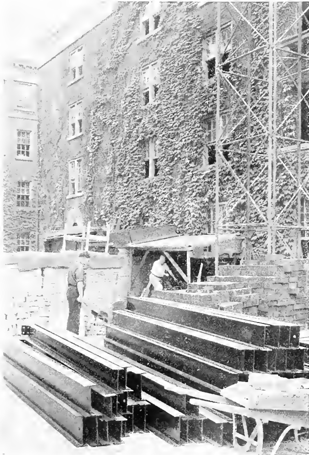
Construction Gets Under Way
